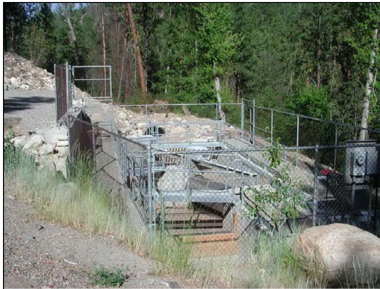
Fish & Wildlife Dept of; Skyline Canal Fish Screen (#00-1158) Attachment #1, New screen
