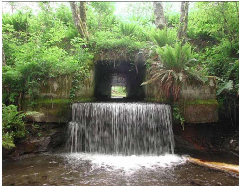
Lewis County Public Works; Lambert Creek Barrier Removal Project (#01-1219) Worksite: #1, Lambert Creek Barrier Removal 06/05/2002, Image #2, Culvert outfall
