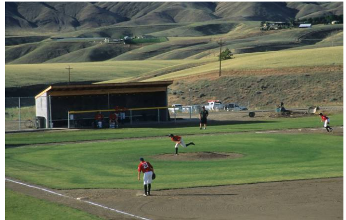
Asotin County Little League used a $147,000 YAF grant to develop three baseball fields, a parking lot, and a building complete with restrooms, concessions, and office space.
