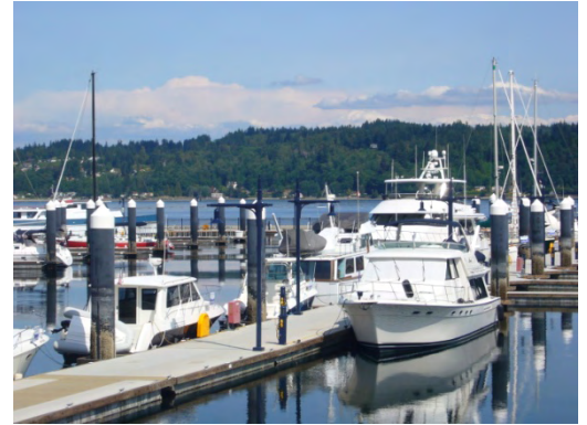
The City of Bremerton used a $950,000 Boating Infrastructure Grant to build a breakwater to enclose the marina and protect it from wakes, and to more than double the guest moorage.
